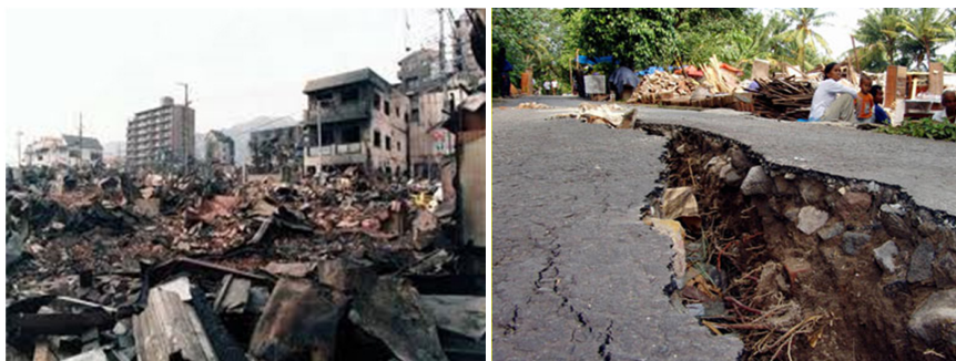
Fig. 30.3 Collapsing of buildings and build up debris
